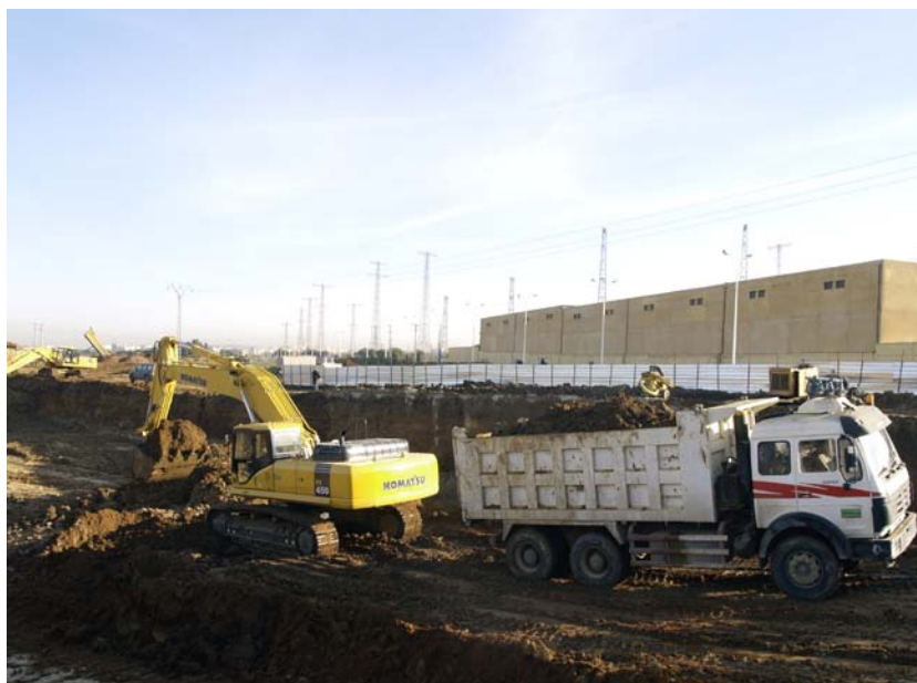
construction of a road in Algiers suburb
