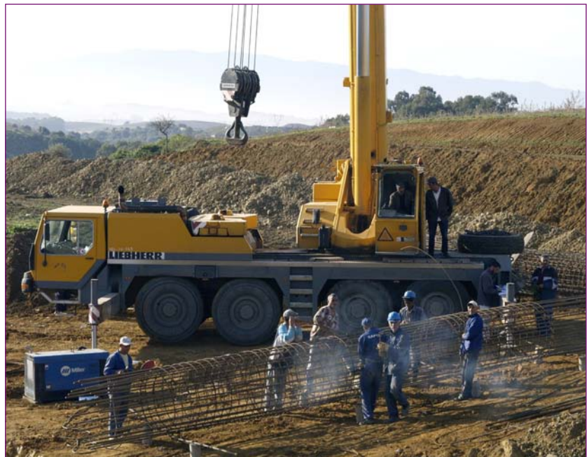
construction of the East-West Highway ( 1200 kms)
