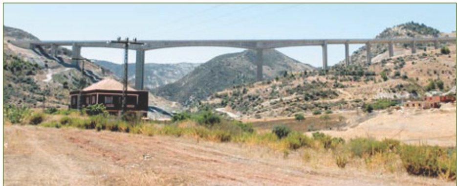
Realising a viaduct on the East-West Highway near Lakhdaria (Bouira Wilayate/prefecture)
